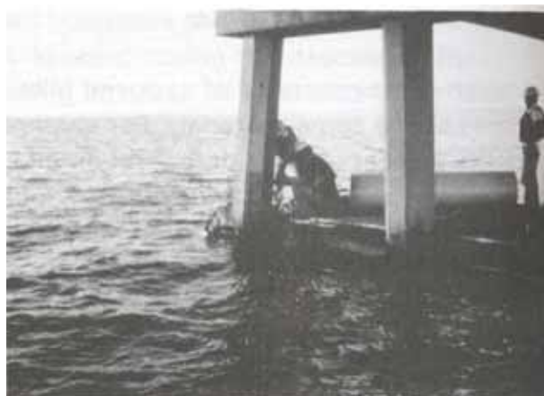
Exhibit XII.11 Installing Pile Jacket
